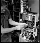
Make any adjustments as needed for proper combustion and wait for analyzer to display any change in the readings. (repeat if necessary)
