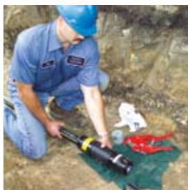
Permasert couplings simplify repairing damaged service lines.
