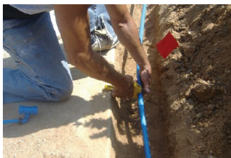
2. Cut-into the lateral line
