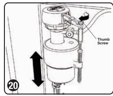
A Thumb Screw is provided to fine-tune adjustments to float. Proper water level should be indicated inside tank or 1/2" to 1" (13 - 25 mm) below overflow tube.
