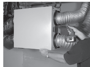
Fix and secure with four screws supplied and seal all joints.
