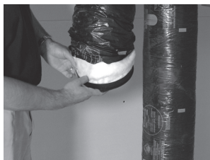
Insert insulation inside the double collar.
