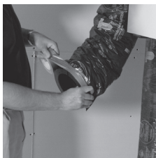
Finish by taping the vapor barrier to the collar to ensure proper seal.
