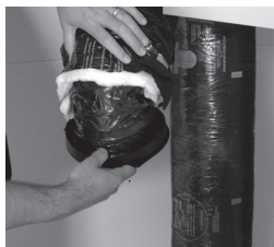
Insert vinyl duct over the hooks and seal with a Tie wrap
