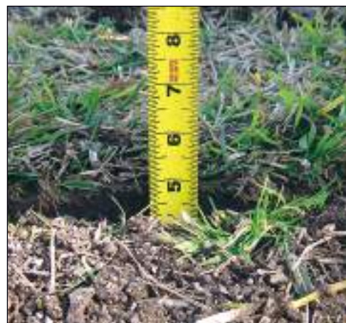
Ensure that dripline depth is consistent throughout the installation
